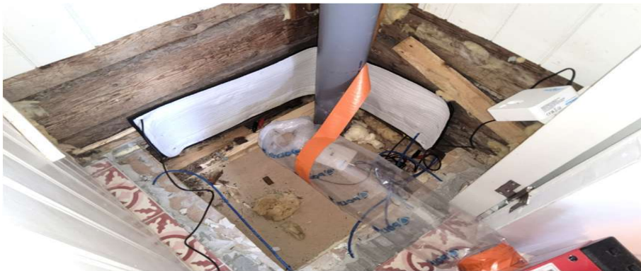
InfraVivo IR Drying Blanket - field test in a Bathroom
