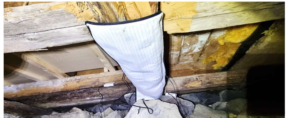
InfraVivo IR Drying Blanket - Feldtest an Blockwand
