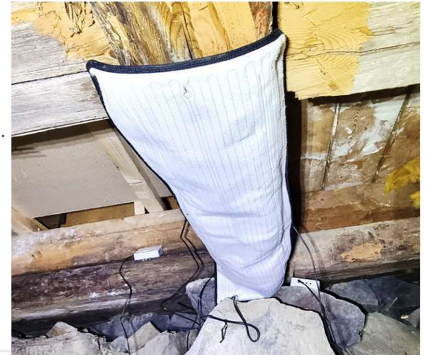
InfraVivo IR Drying Blanket - Feldtest an Blockwand
